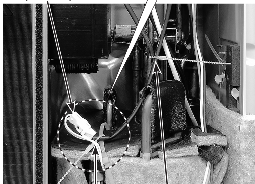
B Connector of the compressor protector
