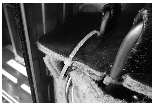
Add the fixing band through the hole for the discharge pipe.
