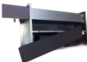
Retirer le bloc mousse anti- condensation
