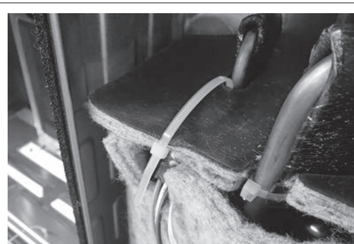
Add the fixing band through the hole for the discharge pipe.
