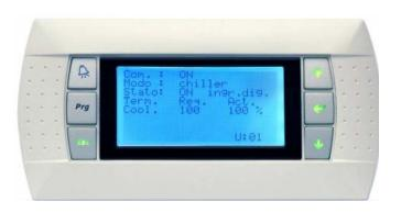
Display and acquisition of the last 200 alarm events (user level) are also available as well as recording of operating variables in the 10 minutes prior to each alarm event (assistance level through Black Box) with display via PC. Compatibility with remote keypad (management of up to 8 units).
